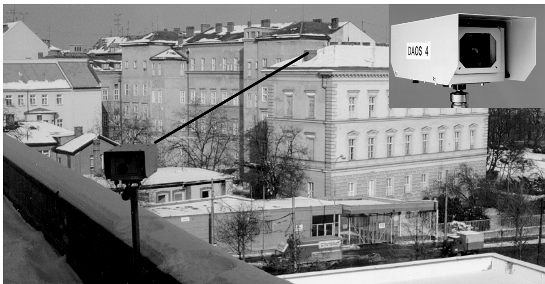
Fig.3. Digital atmospheric optical link between two Hospitals and design of the DAOL head (in the upper right-hand part of the picture).
